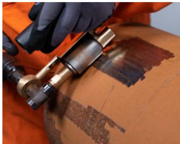
Spot repaired surface on pipeline
